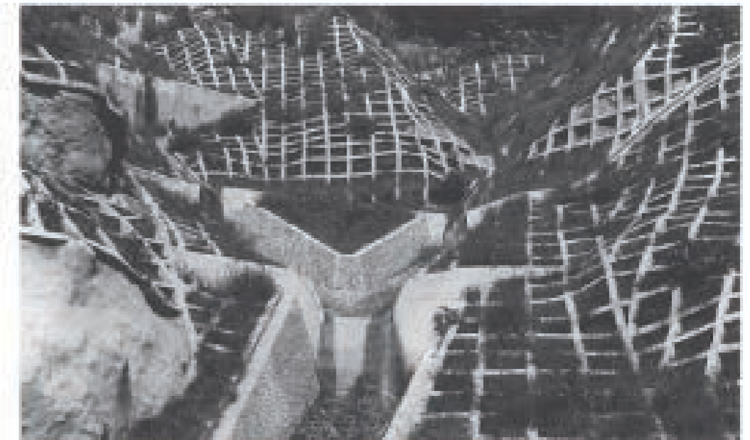
Reference: bank reinforcing structure
