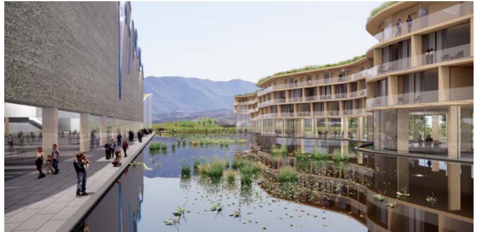
View of Recycled Grey Water System Pond, Expo Albania
