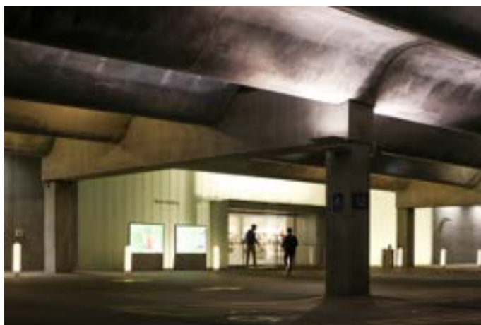
Nelson Atkins Museum of Art, basement opening Steven Holl Architects
