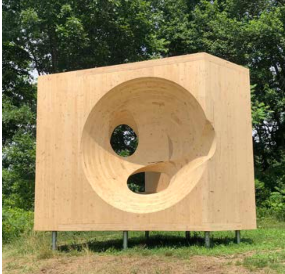
"Obolin," located at the Art Omi Sculpture and Architecture Park in upstate New York was fabricated from on sheet of CLT using a 7-axis robotic arm. The sculpture marks the exact locations of the sun during the Equinox and Summer and Winter Solstices. The materiality is the same as our proposed Wine Hotel.
