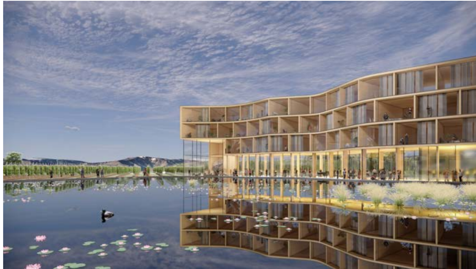
Wine Hotel and Central Landscape Pool Connected to Recycled Grey Water System
