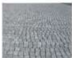
Granite Stone Setts - FF2 Colour: silver grey, material and colour to match adjacent pavers. Finish: flamed Nominal Size: 100 x 100 x 100 mm Joint width: 6mm nominal
