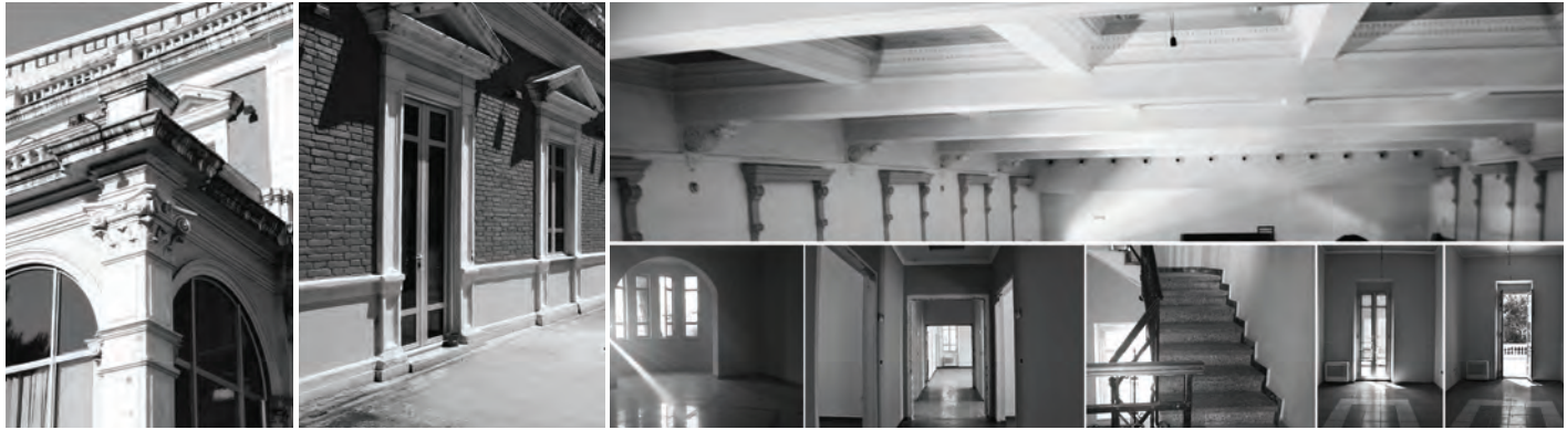
Building existing state
